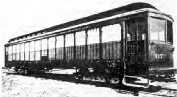
THIS IS THE WAY IT LOOKED WHEN RAIN THREATENED
